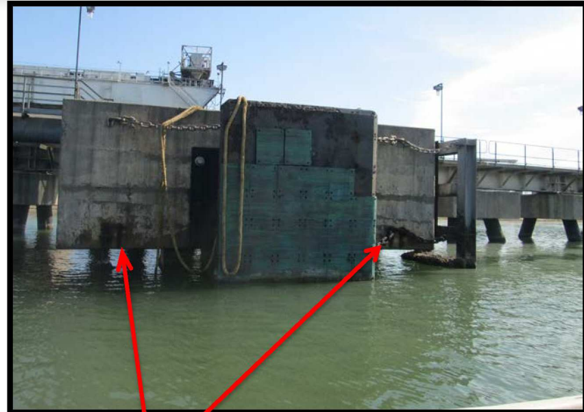
Repair various concrete cracks and spalls
